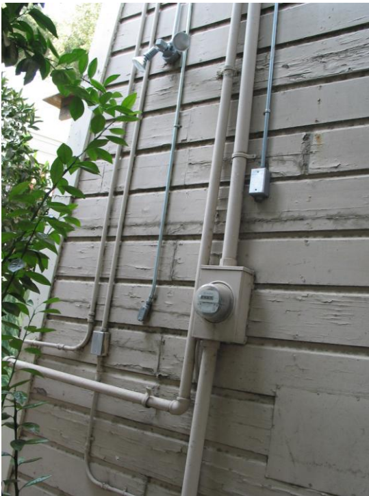
Siding penetrations and conduit
