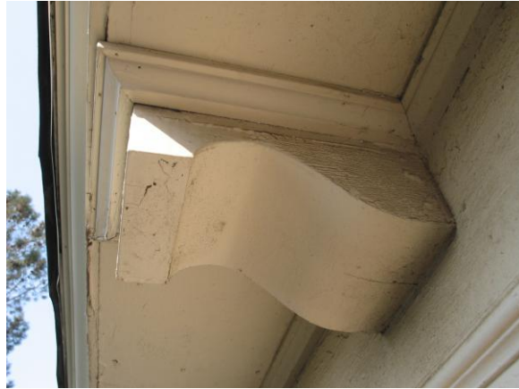
Beam under fascia. Wood appears to be solid.
