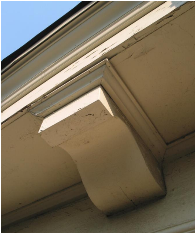
Existing Fascia and fascia beam
