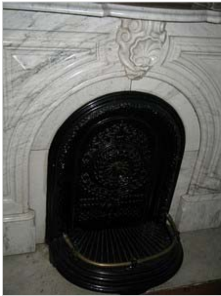
Marble Fireplace with cast iron stove insert - One of Four
