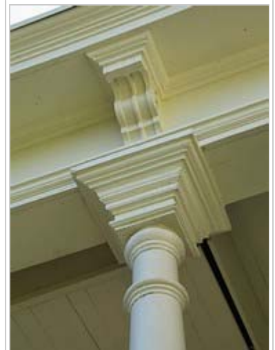
Gingerbread - Porch Post and Cornice Bracket
