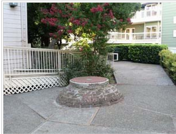
The Brick Soft Water Cistern - E Street side of mansion near back door & ADA ramp, Mansion Square in background
