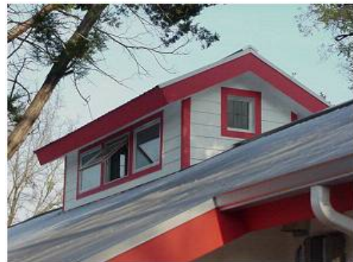
Figure 1. Roof monitor or cupola 1
