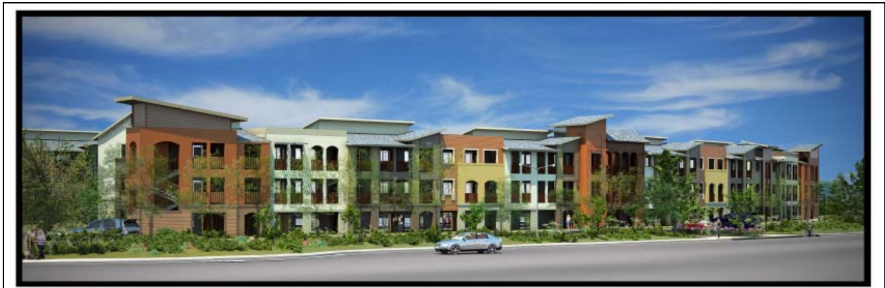
Figure 8. North Elevation View of Building “B” from Cowell Blvd.
