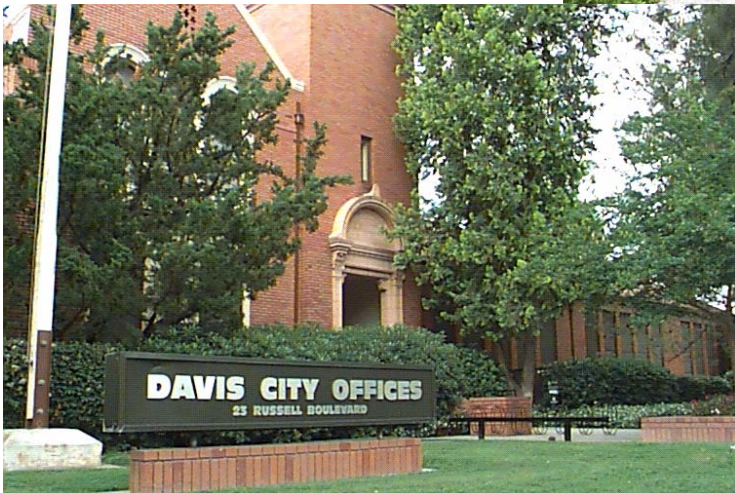
Pictures of Davis City Hall located at 23 Russell Blvd.
