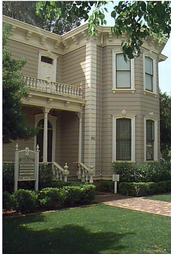
Hunt Boyer Mansion located at 604 2 nd street.
