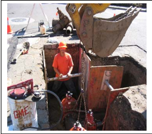
Replacement of 3 mainline valves at Spruce Lane and Claremont Drive
