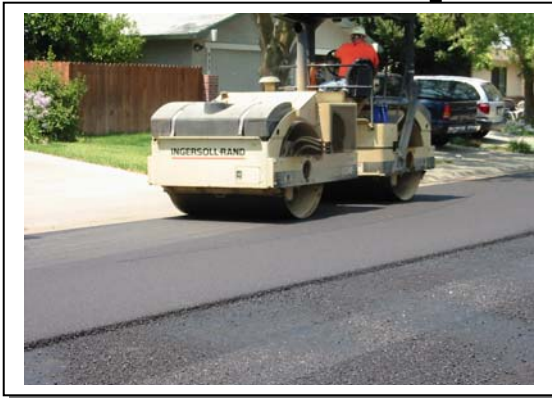
Asphalt concrete overlay.
