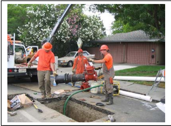
Mainline valve replacement Radcliffe @ Orange.
