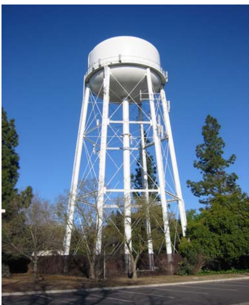
Elevated Water Tank
