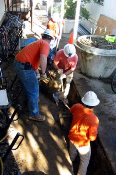
Installing sewer line for new modular unit at Corp. Yard.
