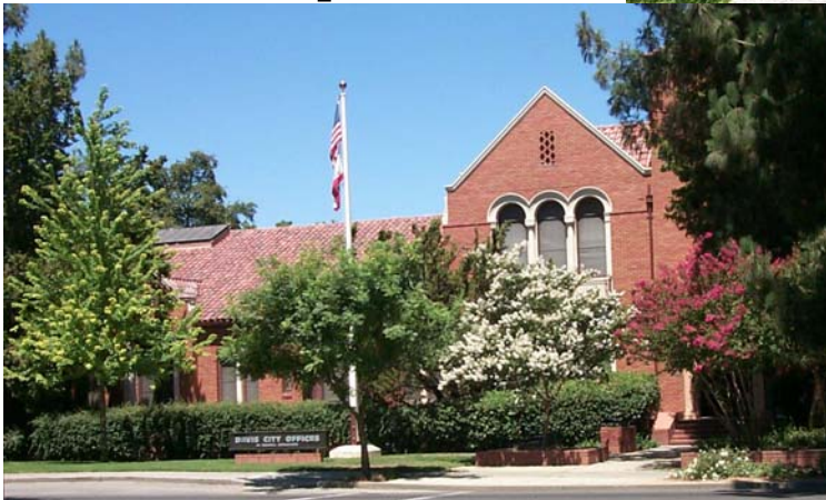
Pictures of Davis City Hall located at 23 Russell Blvd.
