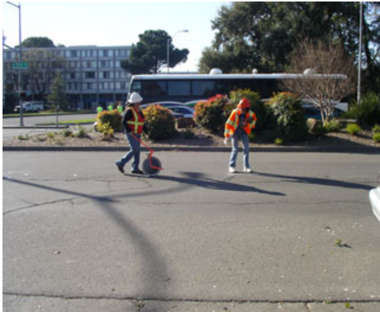
Measuring Russell for Overlay Project
