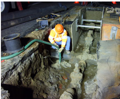
4th @ F Street Water Main Valve Replacement
