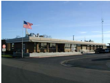
Wastewater Treatment Plant
