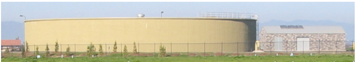
West Area Tank
