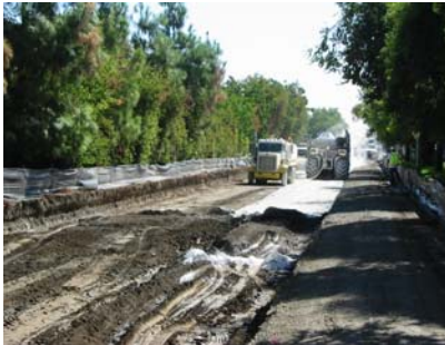
Covell Subsidence Repair
