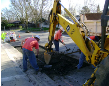
Catalina & Anza Asphalt Replacement
