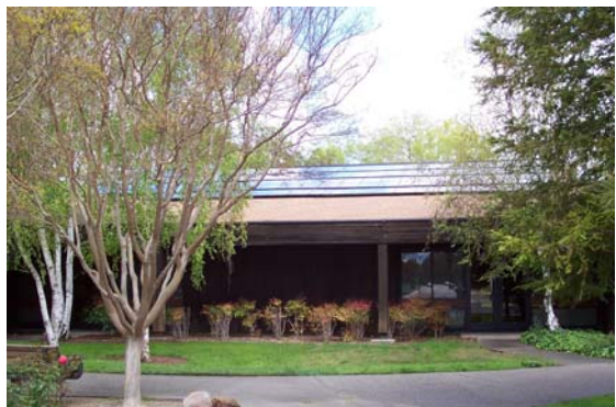
VMC Solar Panels
