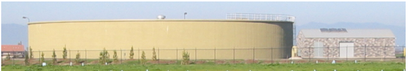
West Area Tank
