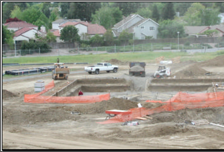
Arroyo Park Pool
