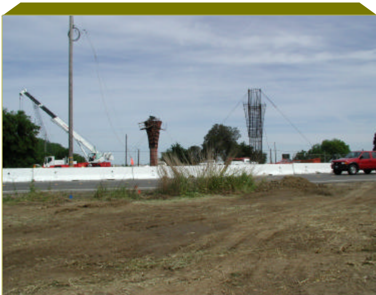
Dave Pelz Bicycle Overcrossing
