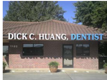
Unacceptable Signage: Sign scale is not appropriate for the building
