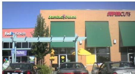
Unacceptable signage: Multiple tenant wall signs along a building's façade should be mounted along the same plane and should be located closer to storefront opening
