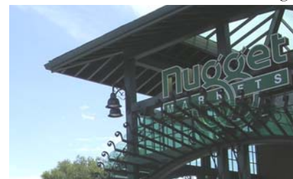
Sign is well integrated with building’s architectural features
