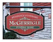
Mounting hardware should be an attractive and integral part of the sign design. Simple round pipe brackets with plugged ends or added decorative end elements are generally appropriate for signs. However, metal brackets of a more decorative and complex shape are encouraged where appropriate to add to the character of the building.
