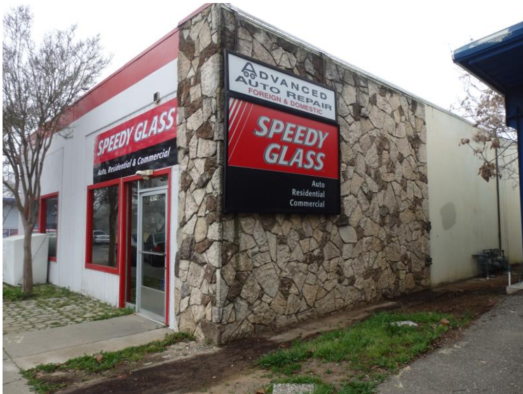
Photo 12 Bldg. 9-965A West Olive Drive.
