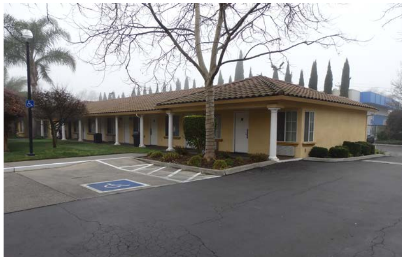
Figure 3. Building 4 constructed 1956; remodeled 1997. Facing south.
