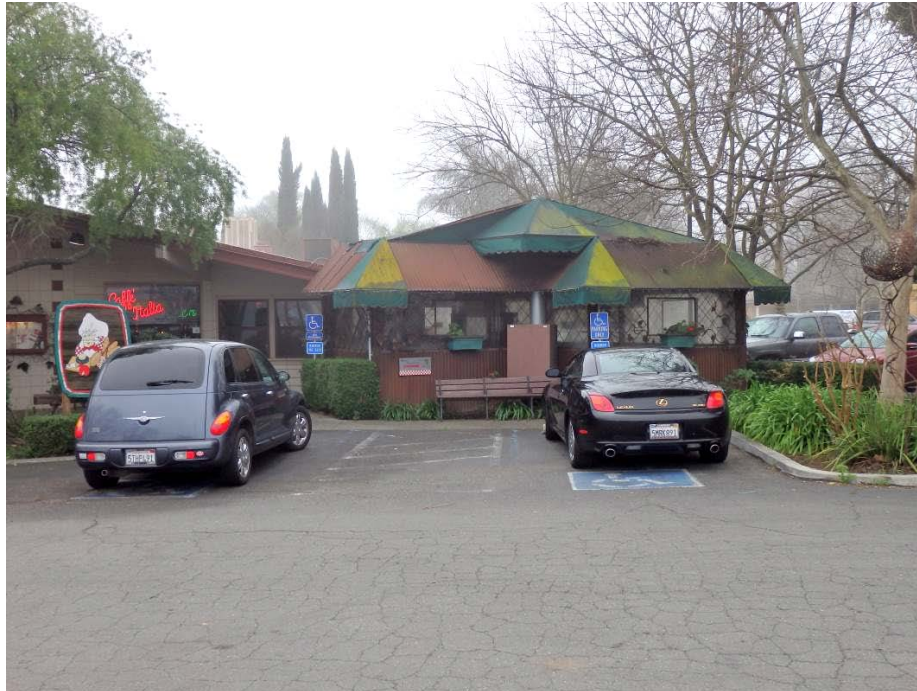
Figure 2. Looking southwest, view of covered patio.
