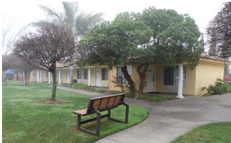
Figure 4. Building 5 constructed 1959; remodeled 1997. Facing south.
