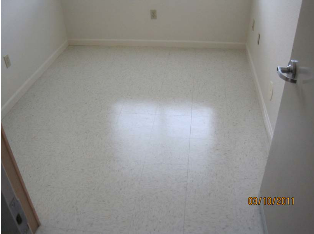
Vacant rooms “after” work by YCH –
