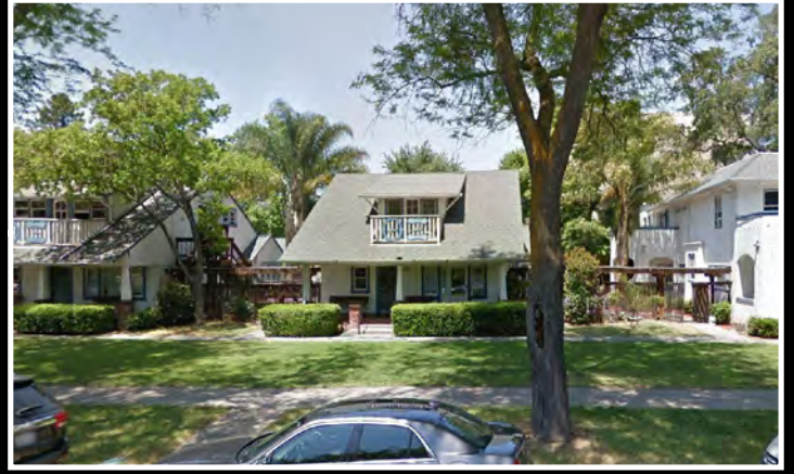
View north on First Street - Bryson House
