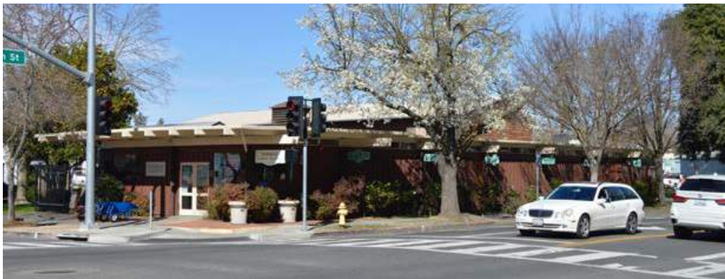
Figure 5.20 Hibbert Lumber Company building
