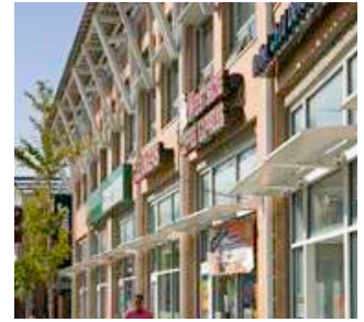
Figure 3.22 Green Building Green building features are integrated into the building facade.
