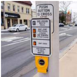
Figure 6.18 Audio Crosswalks Universal Design features such as tactile crosswalk materials (above) and audio crosswalks (below), can easily be integrated into street design at little additional cost.
