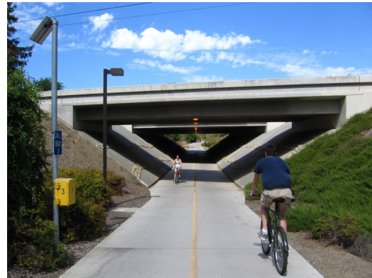
Figure 11: Putah Creek undercrossing. Photo: Philip Neustrom
