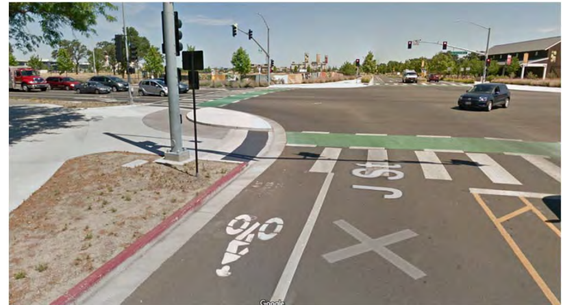
Covell Boulevard/J Street Davis, CA
