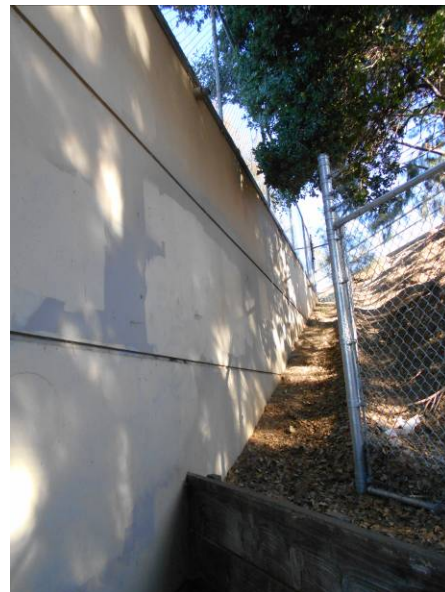
Embankment against structure.
