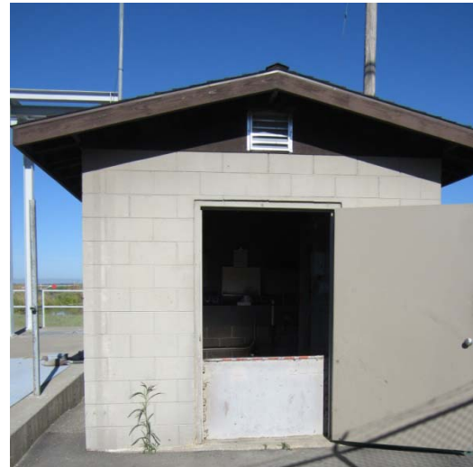
Plate across building door
