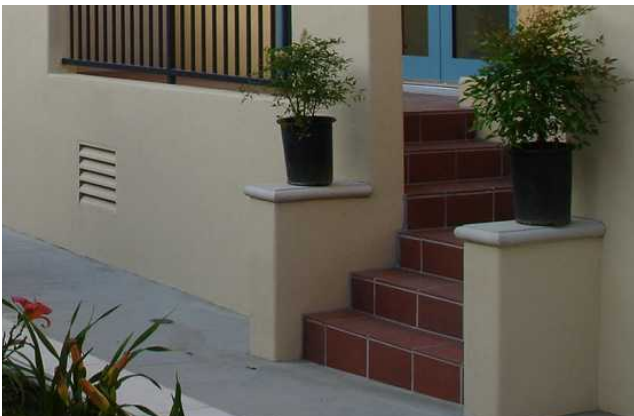
Stoops define the entry to this dwelling while elevating the ground floor from the sidewalk level.
