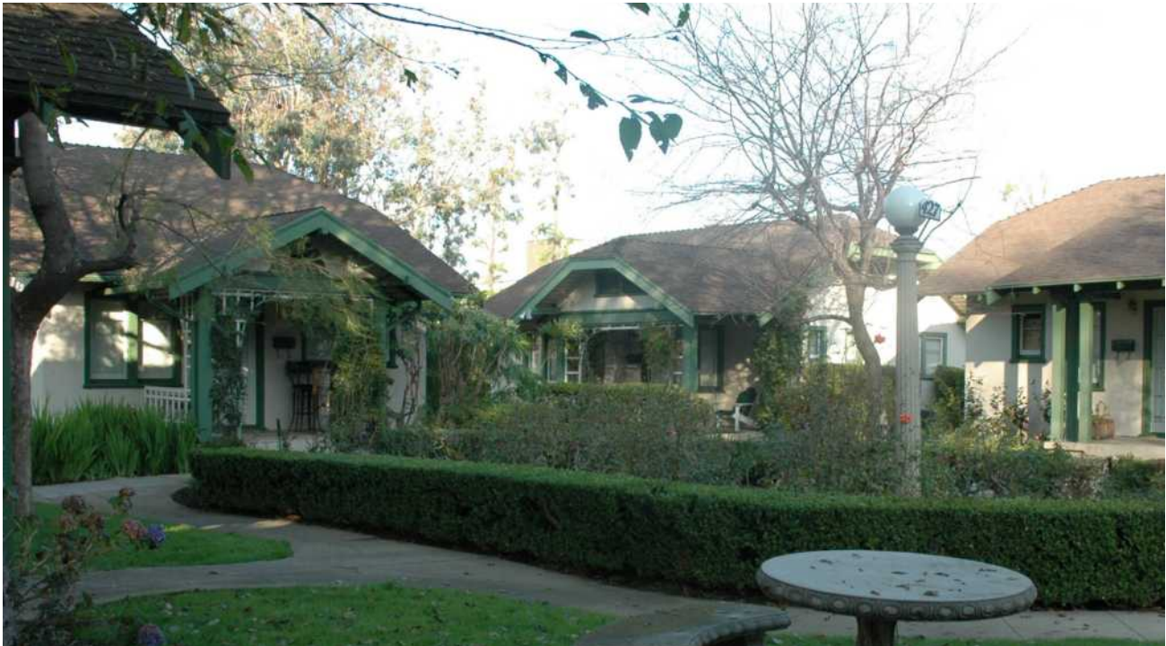
A five-building, one-story Cottage Court with projecting porches along a court leading to entries.
