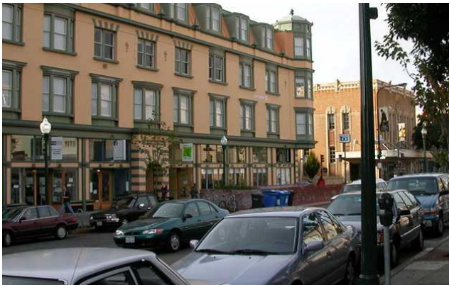
Three-story Main Street building with occupied attic space.
