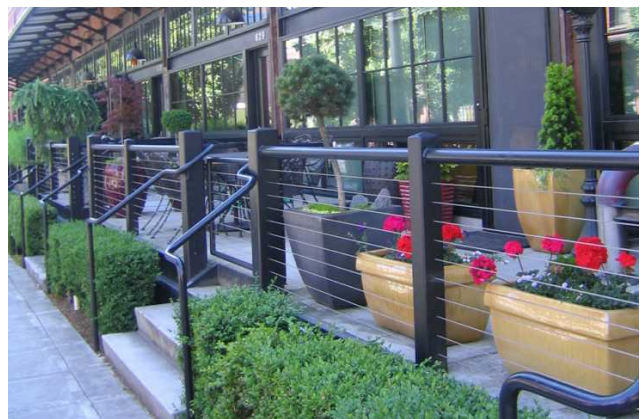
One terrace spans across several ground floor live/work units with individual entries separated by landscaping.
