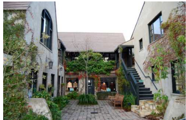
Forecourt visually extends the public realm into this retail and office building
