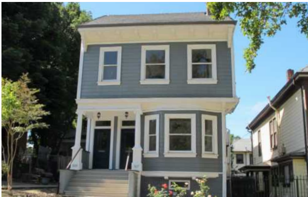
Two-story Duplex with engaged porch.
