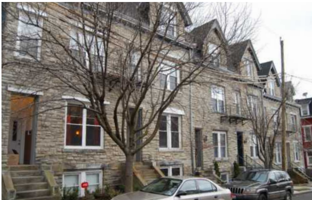
Two-story Townhouses massed as one building.
