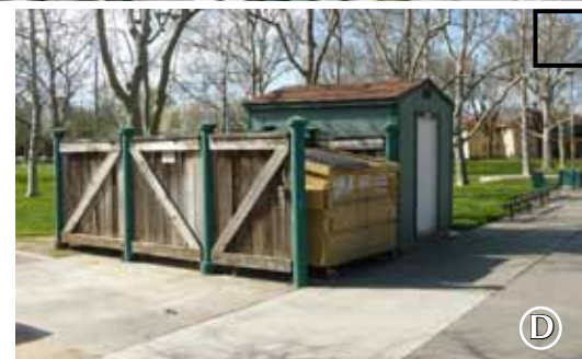
Garbage and storage structure are unattractive and encroach on adjacent walkways.
