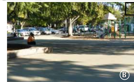
Asphalt area feels barren and unwelcoming. Seatwalls are damaged by skateboard activity.
