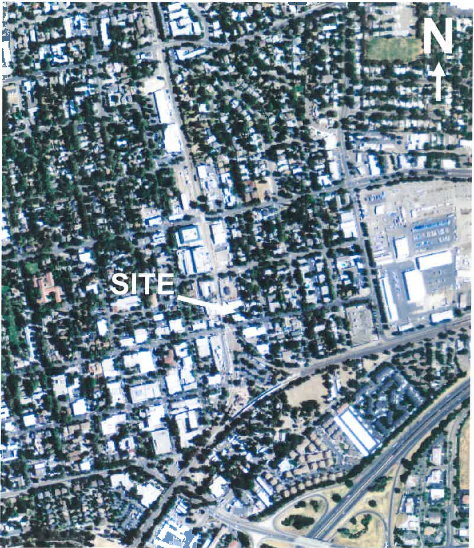
Aerial Photo, 2012: APN 070-324-002, 901-919 Third Street, Davis, CA 95616. Photo shows site containing two retail/commercial buildings.
