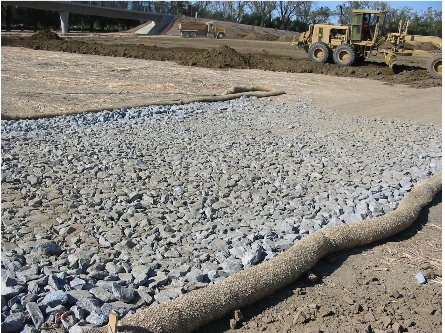
Sediment Control BMPs at Second Street near the Dave Pelz Bike Overcross of I80.
