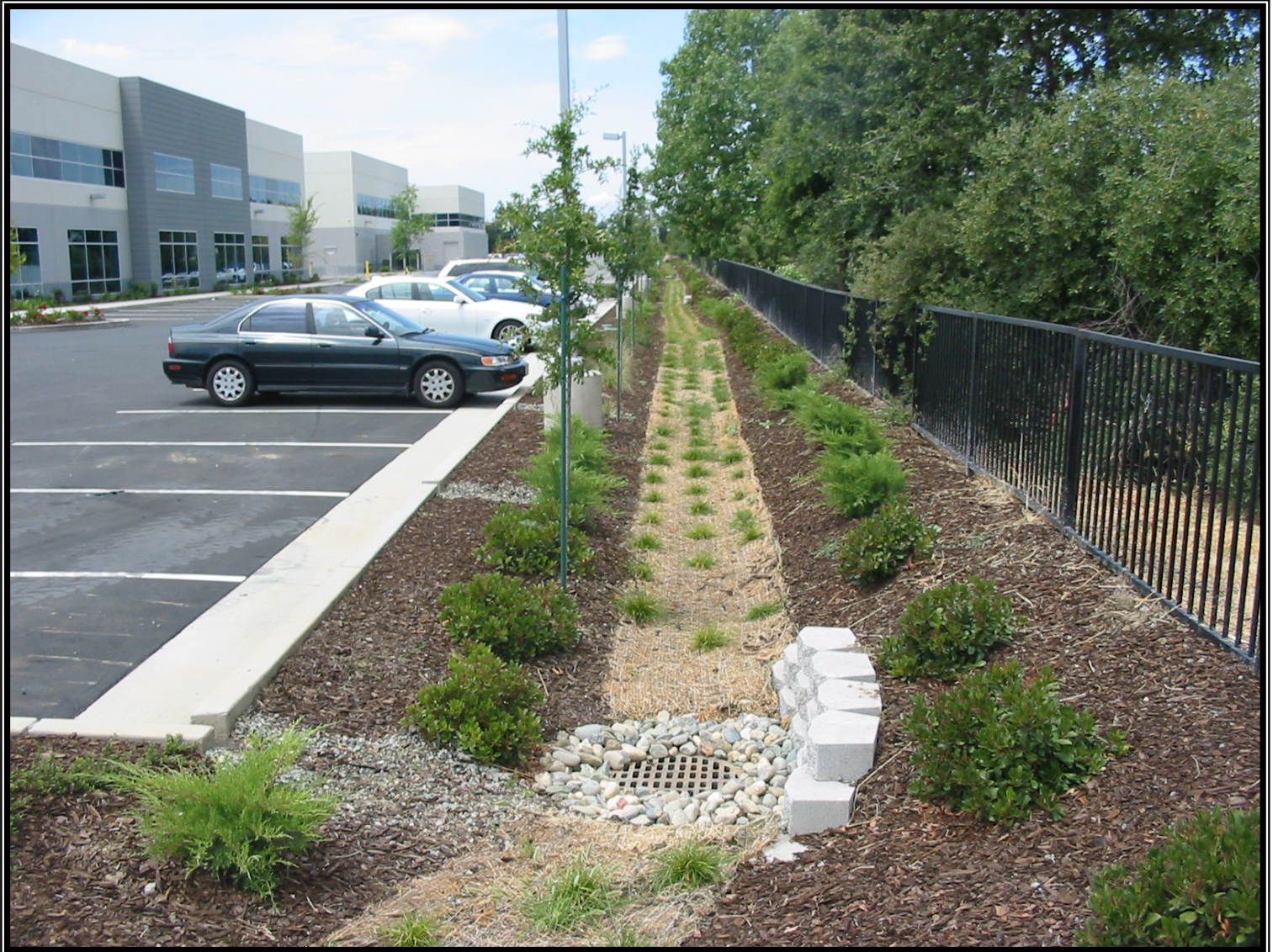
Swale Located on Site at Second Street
