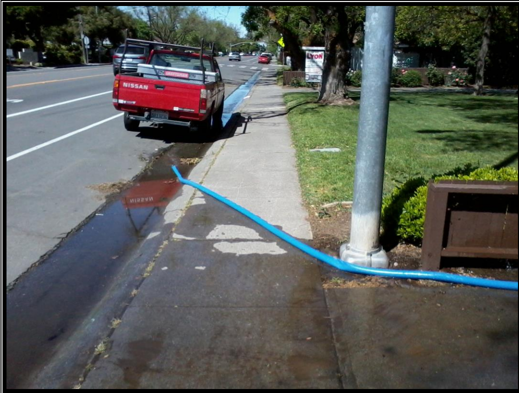
An Illicit Discharge to the Storm Drain System that the City Responded to on Anderson Road.
