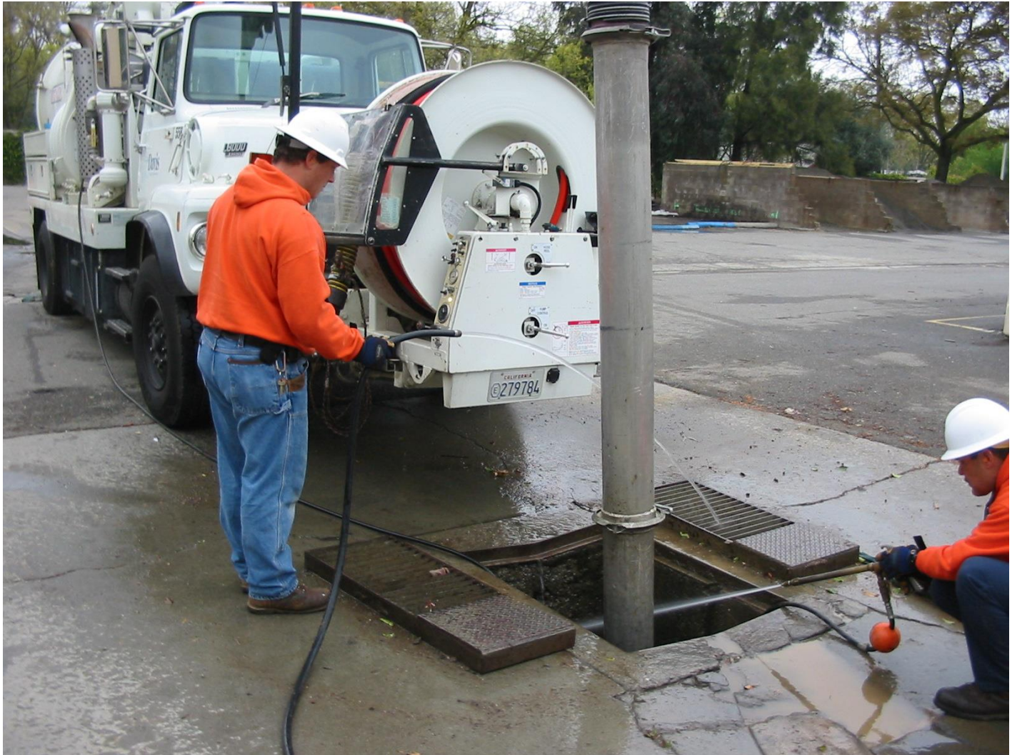
City Crews Vacuuming out a City Storm Drain Inlet
