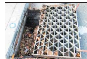
City crews proactively clean clogged drains before storms
