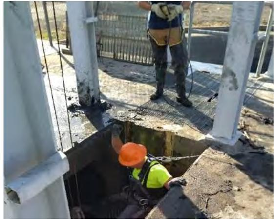
*Staff clearing out dirt and other debris from the pump station wet wells.*
