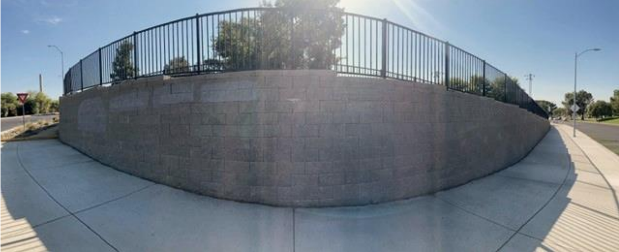
Panoramic of site-- large retaining wall on the southeast corner of F St. and Covell Blvd.:
