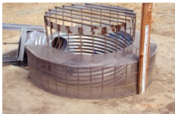
Figure 1 Example of Extended Detention Outlet Structure
