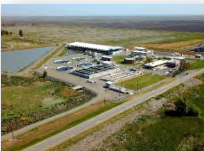
The City of Davis Wastewater Treatment
