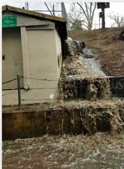
Stormwater drainage station on Richards Blvd during a major storm in 2023
