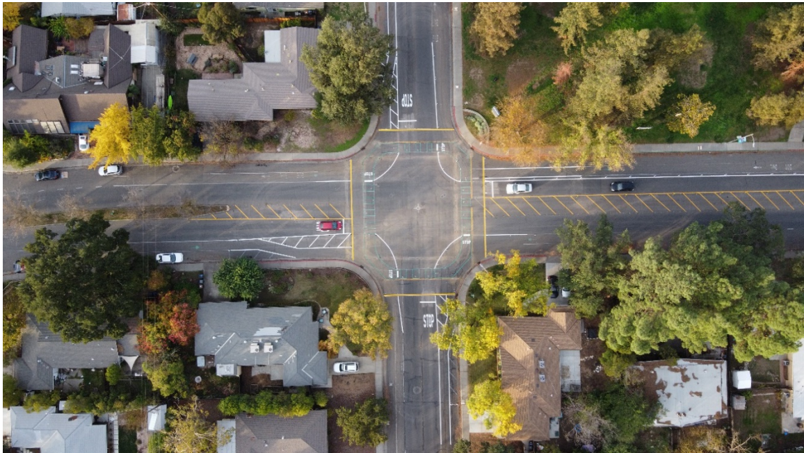
Figure 3: West Fourteenth Street & Oak Avenue Protected Intersection
