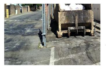
Discolored surfaces usually indicate some kind of pollutants. If you see discolored pavement, do NOT wash these areas off without ensuring that the wash water will go into a sanitary sewer instead of a stormdrain.
