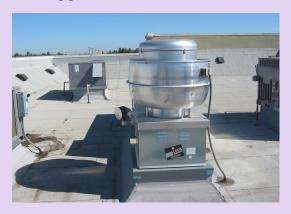
Do not direct dirty water, cleaning solution, rinse water or other material from cleaning exterior exhaust hoods to the roof surface or building gutters.
