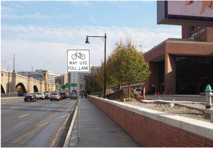
PHOTO: MASSACHUSETTS DOT
