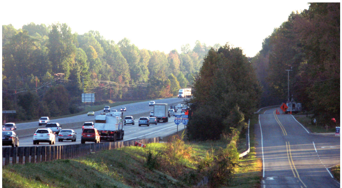
Example of a vegetation barrier along a highway; roadside vegetation barriers have been shown to improve near-road air quality. Questions remain on the optimal design features for effectiveness.
