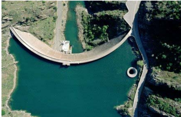
An aerial view shows Monticello Dam and the Glory Hole at right. At the base of the dam, there is a hydroelectric power plant, which generates power mainly for the north San Francisco Bay Area. Construction of the dam began in 1953 and was completed in 1957. It created Lake Berryessa and gets its name from the town of Monticello, which was vacated and then submerged in water as the lake filled up. Solano County Water Agency/Courtesy photo
