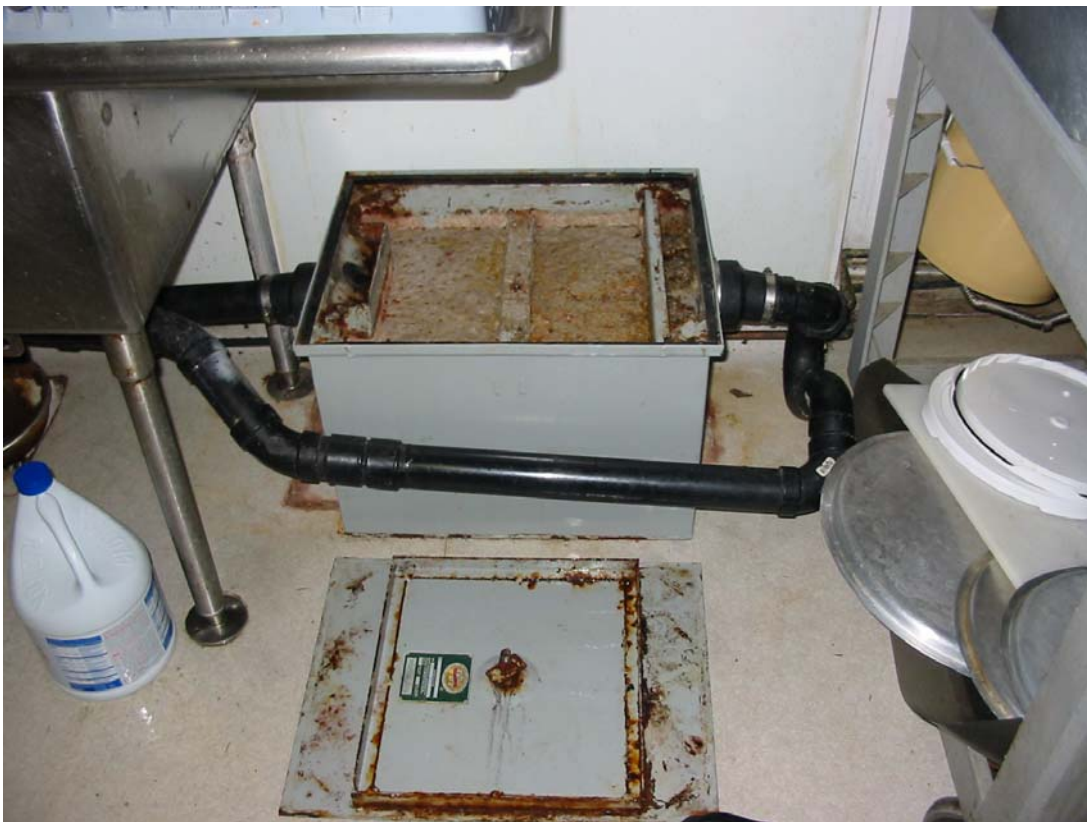
Example of a under counter style grease trap.
