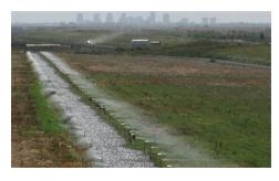
pumps are designed to pump 4,400 G.P.M. Each of the 15 zones has two terraces. Wastewater is evenly distributed over each terrace using spray heads. Each terrace is 150 feet wide with a two percent slope from top to bottom. The hydraulic loading rate is 37,000 gallons per acre per day over the 170-acre field of 15 zones.
