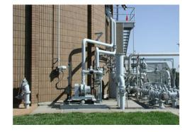
carbon dioxide and 70 percent methane. The digesters are producing an average of 26,000 cubic feet of gas per day, with an average savings in electrical costs of \$100 to \$140 dollars per day.
