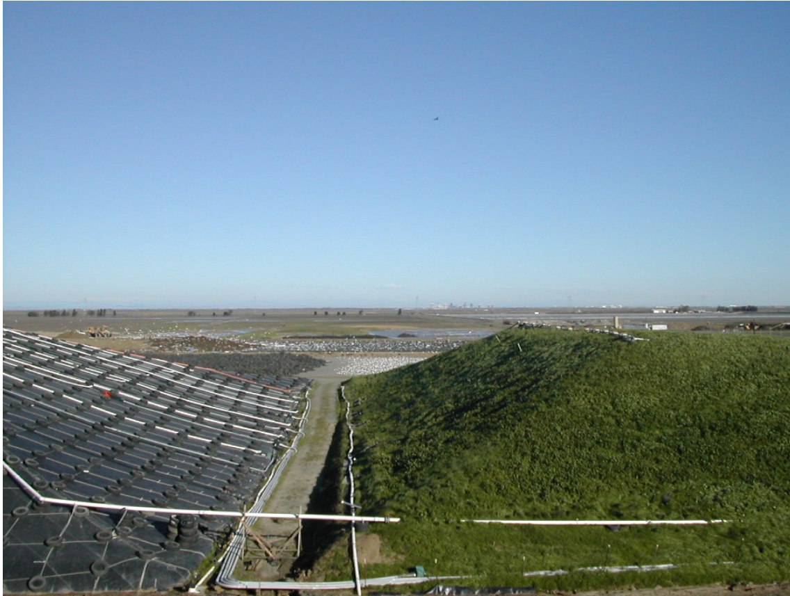
Yolo County Central Landfill
