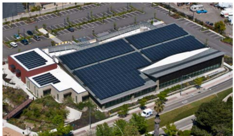
(Photo Courtesy of Sun Light & Power)
