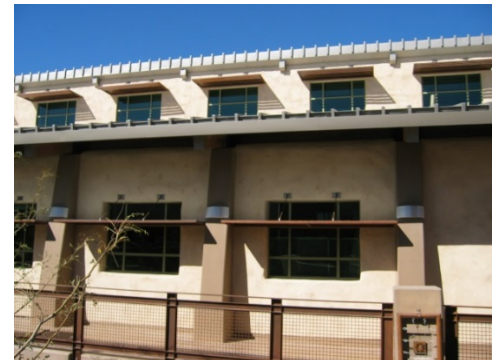
Figure 4-10 Example of Light Shelves in Commercial Building
