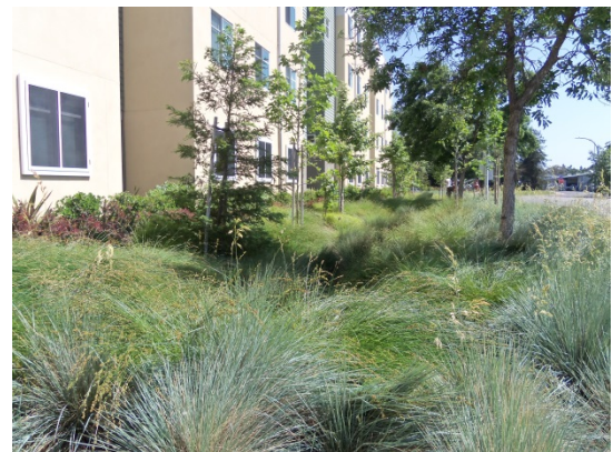
Vegetated swale outside of Tercero II Housing, UC Davis campus, promotes stormwater filtration and infiltration.
