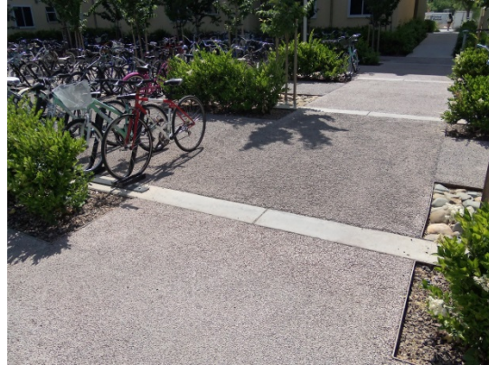
Pervious pavement in a bike parking area allows for a solid surface while still allowing infiltration.
