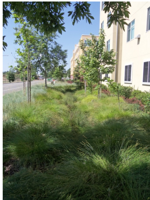
Low impact development techniques include vegetated swales, like this one outside of Tercero 2 Student Housing.
