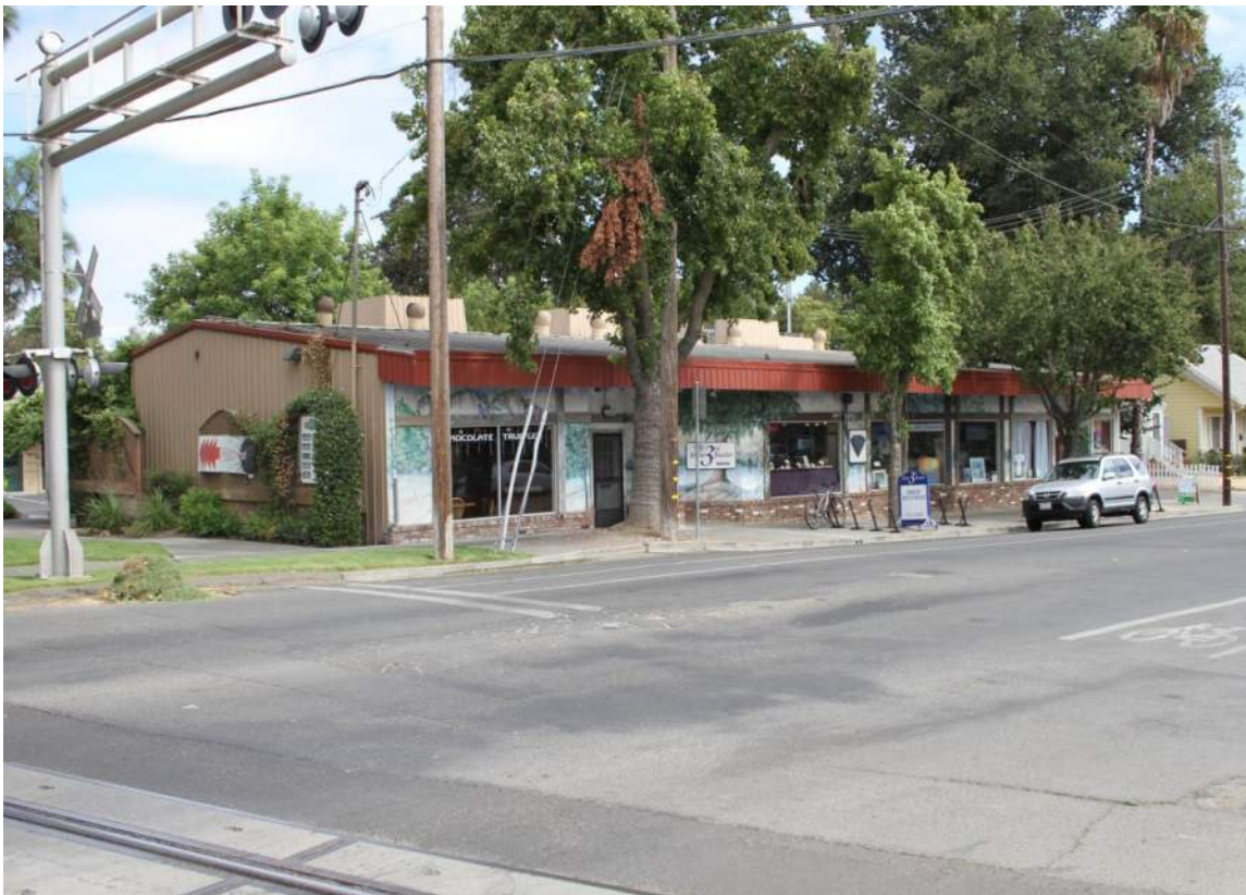
Figure 5. View looking southeast at 901-909 3rd Street, Davis, CA.
