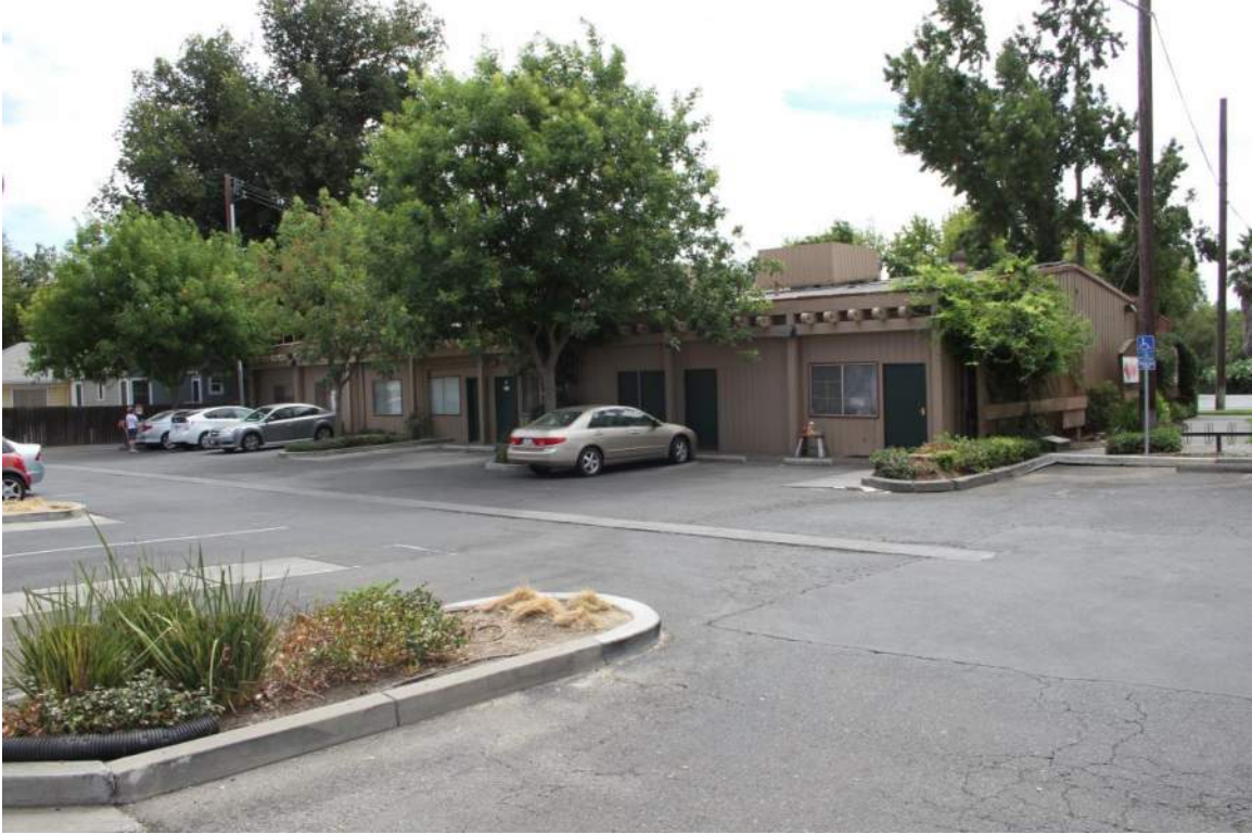
Photograph 15: View looking south at the rear of the westernmost building facing 3rd Street.
