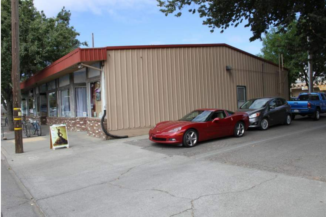
Photograph 7: View of the southeast elevation of the westernmost commercial building, looking northwest.
