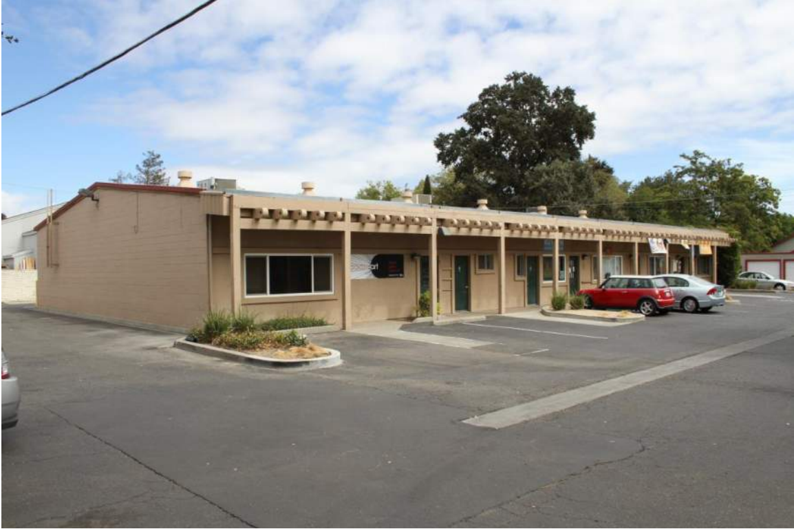
Photograph 13: View looking east at the front facade or west facade of the former motel.
