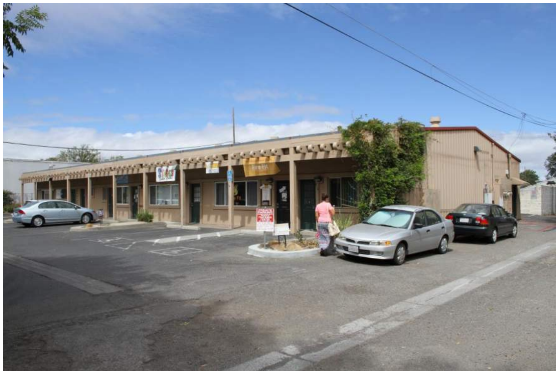
Photograph 8: View looking northwest at the easternmost building on the project site, formerly a motel.
