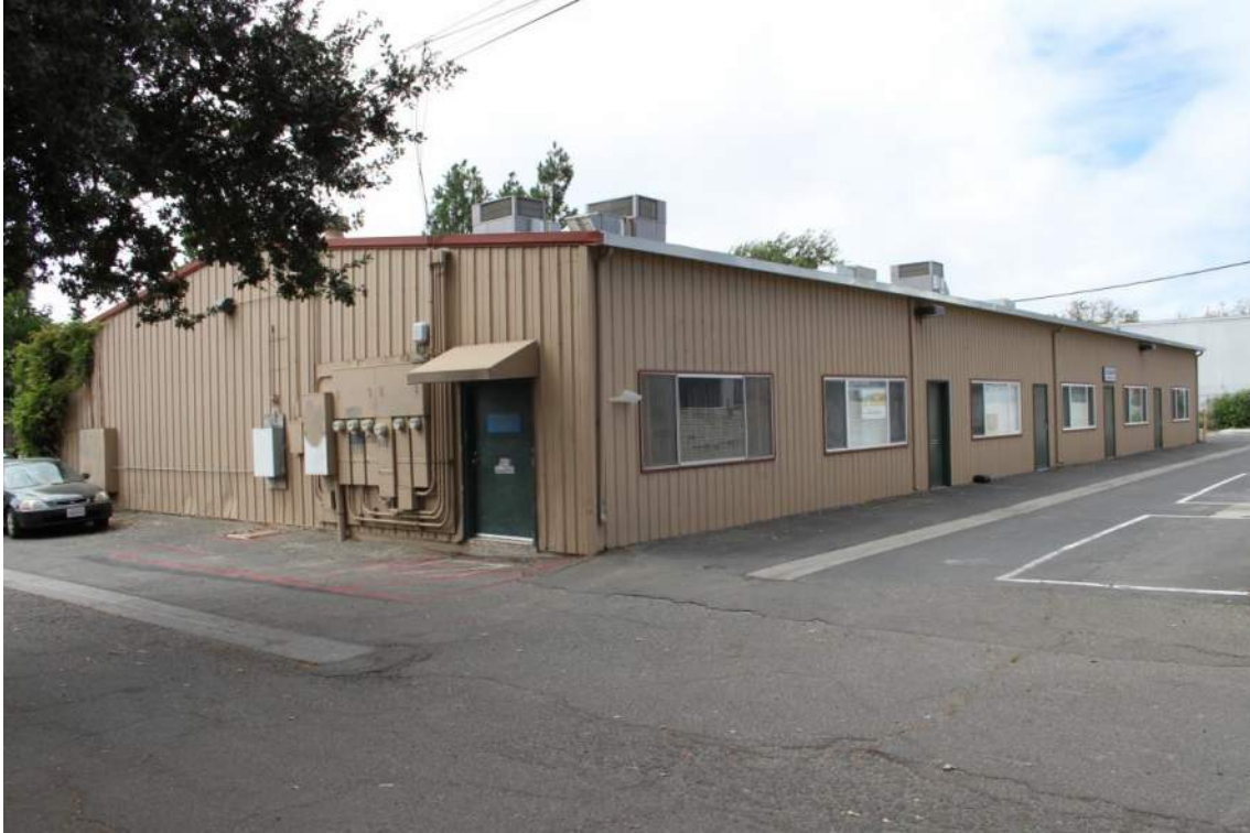
Photograph 9: View looking west at the rear of the former motel. Note the contemporary metal siding.
