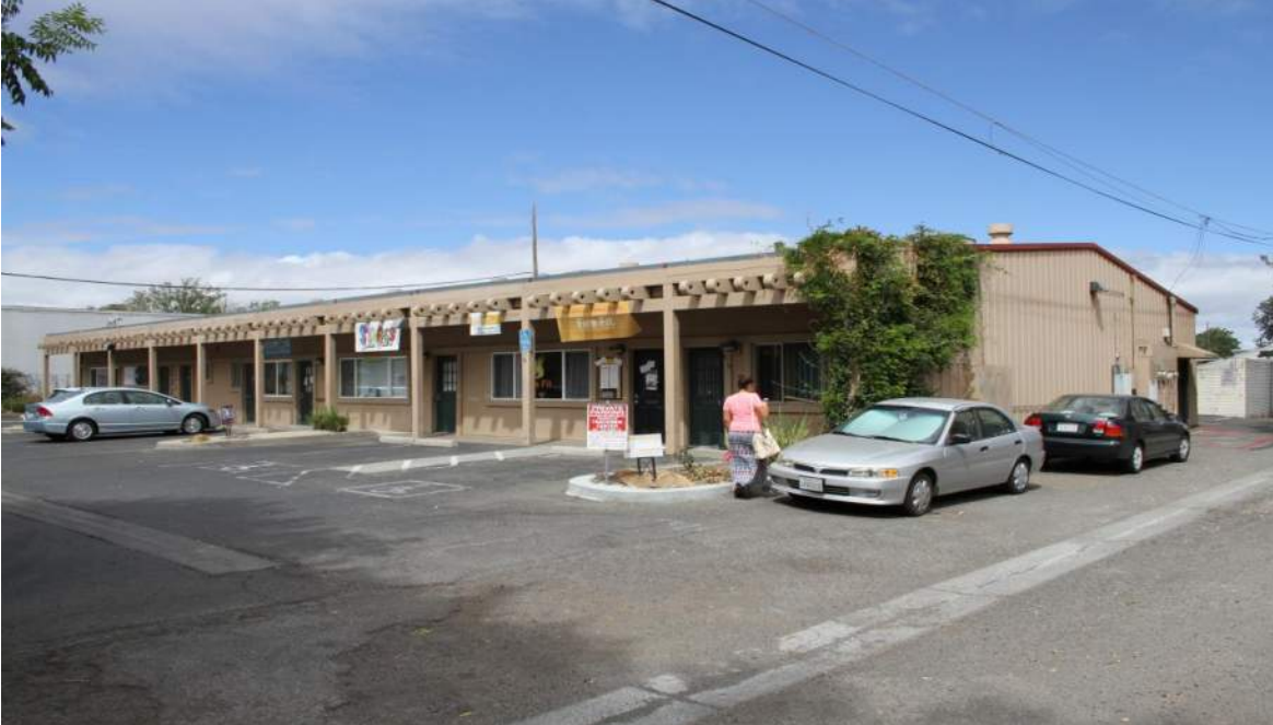
Figure 6. View looking northeast at 911-919 3rd Street, Davis, CA.
