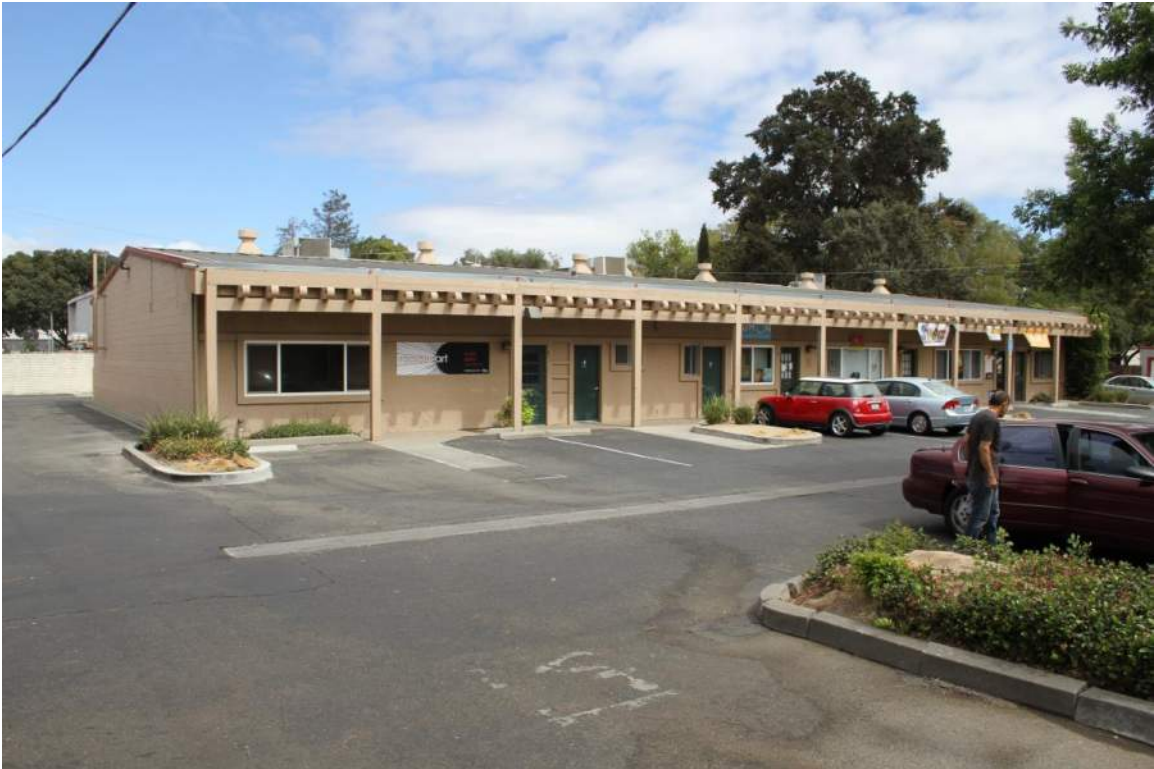
Photograph 14: Another view looking east at the former motel on the project site.
