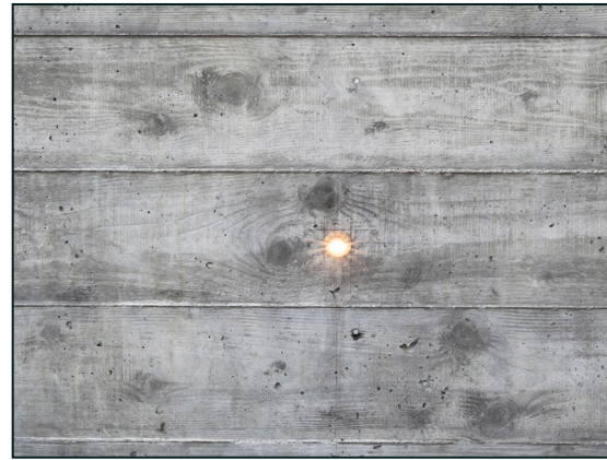
Board Formed Concrete
