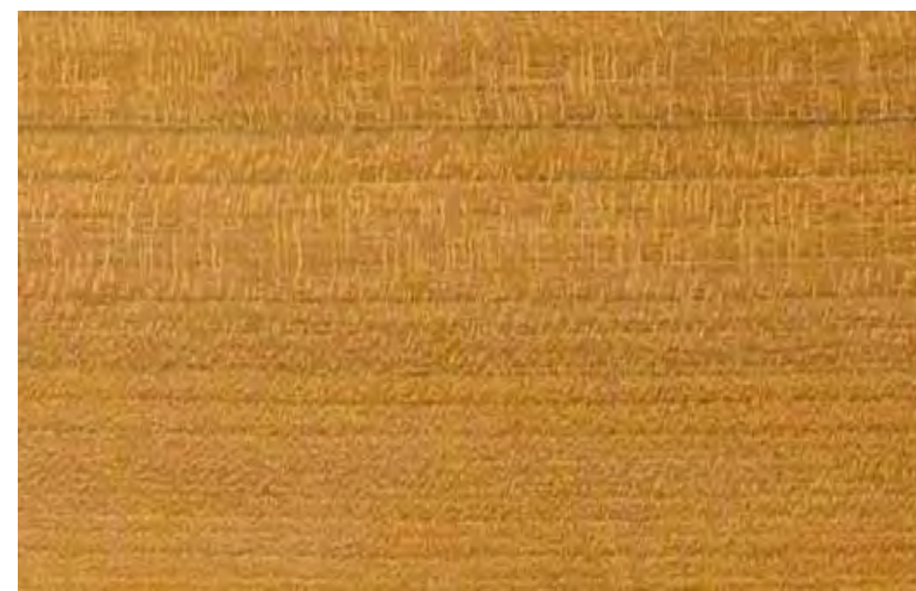
STAINED WOOD TRIM AND TRELIS (EAST SIDE OF BUILDING)
