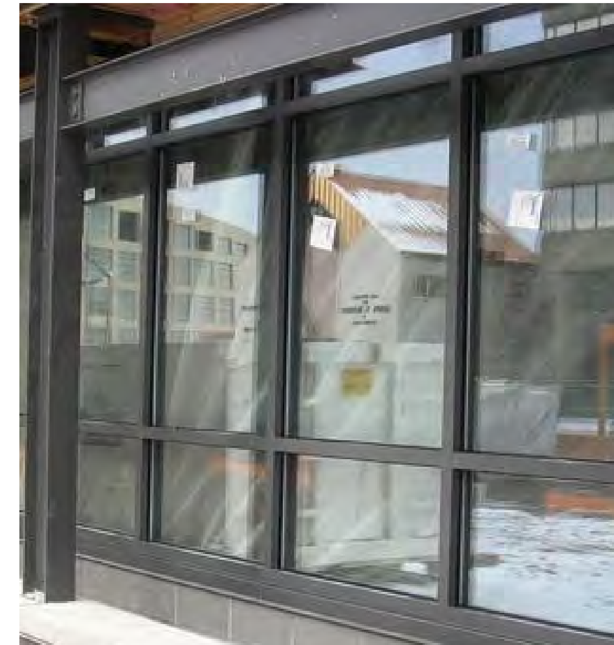
ANODIZED ALUMINUM STOREFRONT / PAINTED STEEL TRIM
