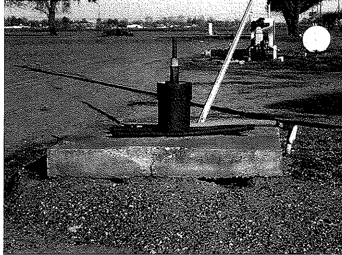
Well pad near Zamora. The pad appears to be fixed to the well casing, while the adjacent ground surface appears to have subsided.
