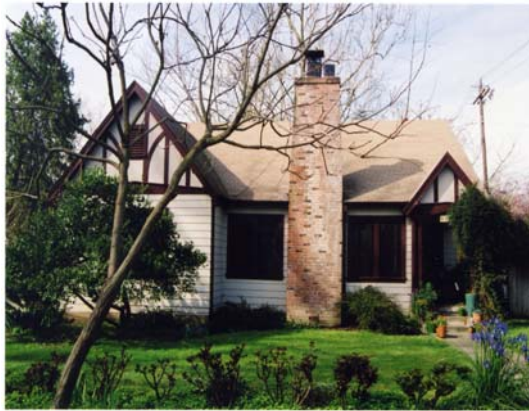
Figure 16 639 E Street Tudor Revival
