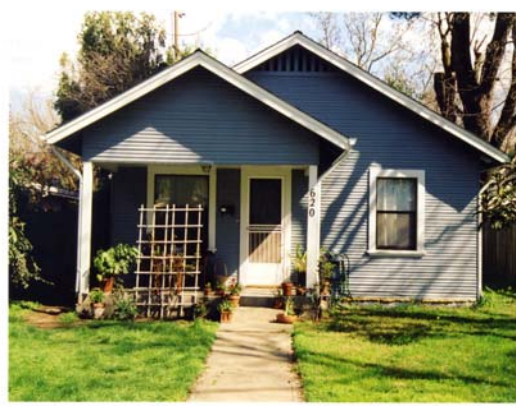
Figure 9 620 F Street Double Gable Bungalow
