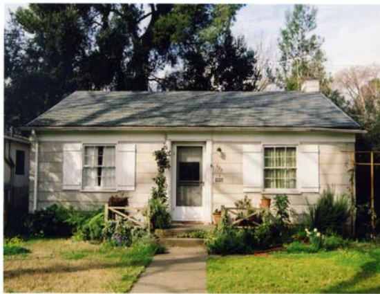
Figure 14 623 C Street Colonial Revival
