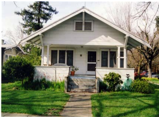
Figure 8 647 F Street Front Gable Bungalow
