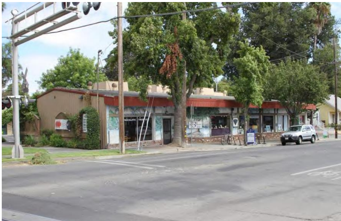
Figure 1.1. View of project site looking southeast
