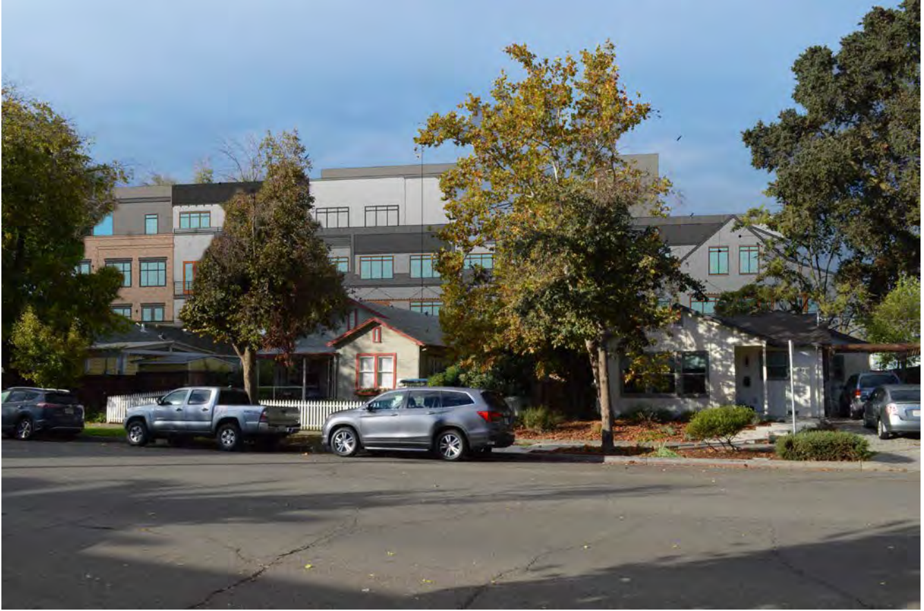
Figure 4: Photo simulation of the proposed Trackside Center building looking south-west from 320 I Street. The simulation was produced by Devin Gumm, a professional graphic designer. A rendering of the Trackside Center eastern facade, produced by the project applicants and available at the City of Davis project website, was superimposed on a photograph taken in October, 2016. The measured heights of existing structures, along with the building dimensions of the Trackside Center, were used to properly scale the proposed building in the landscape.
